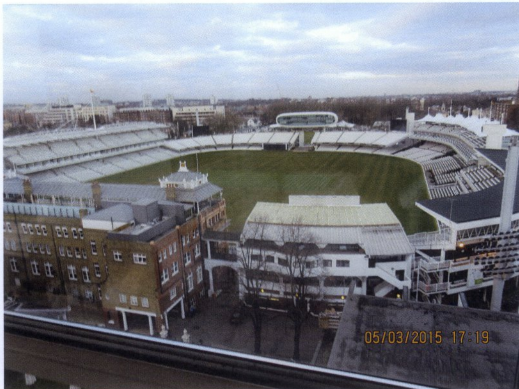
View from Century Court of the rear of the listed pavilion, Allen and Tavern Stands
